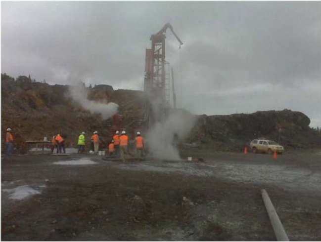
FIG 8 - Drilling operations utilising the conventional cyclone and three-tiered splitter system.
